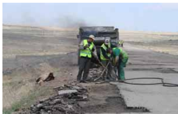
Rehabilitation works on H17 Armavir-Isahakyan-Gyumri road
