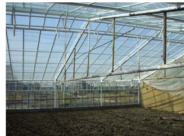
Renovation of the greenhouse is ongoing
