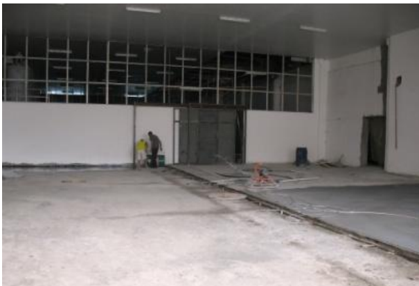
Fruit sorting centre is under renovation.
