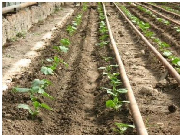
Pipes of heating system are already installed.
